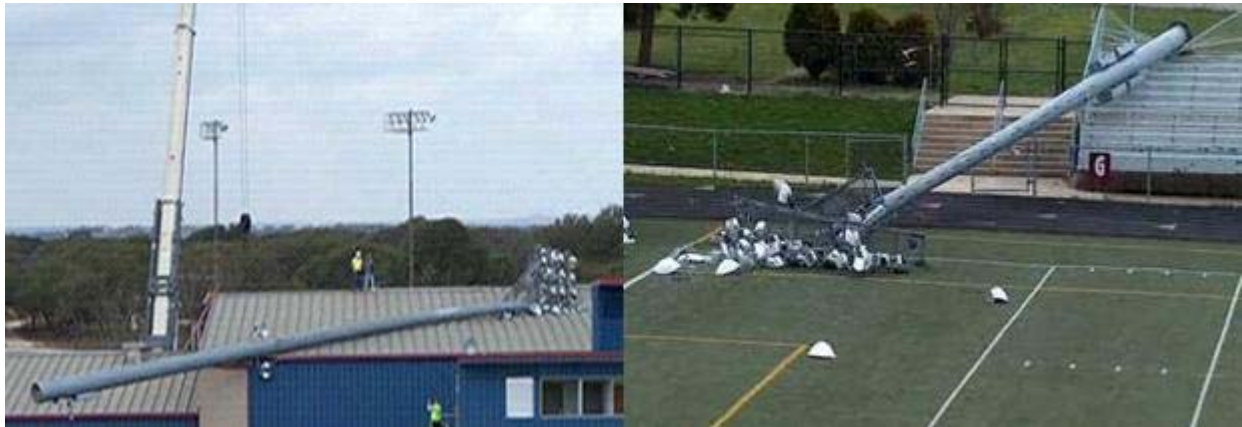
Fallen Stadium Light Poles
