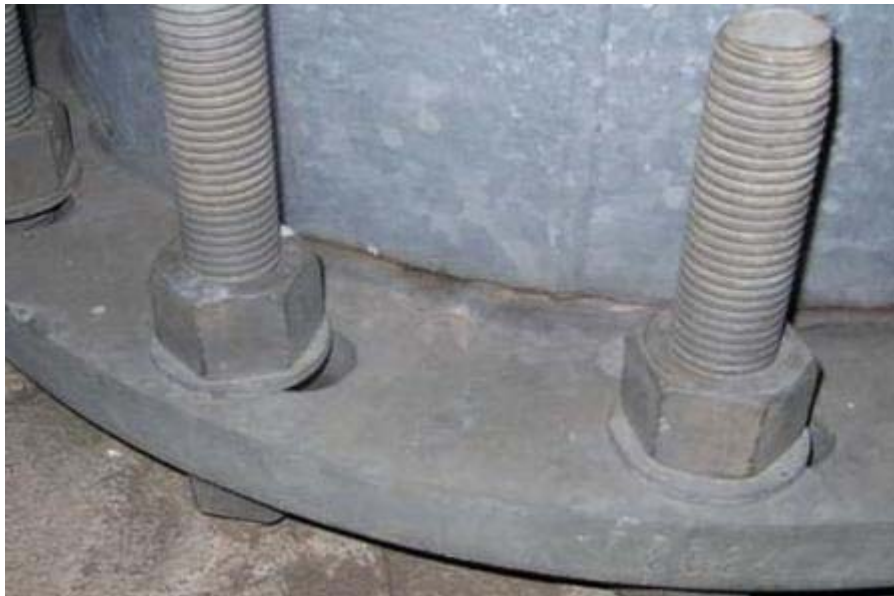
Base Plate of Stadium Light Pole
