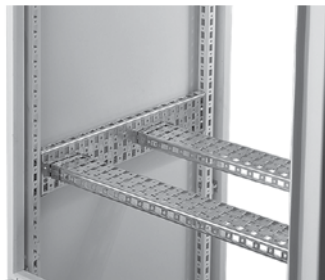
Grid Strap installation (side to side)
