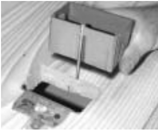
Install clip over subfloor.
