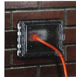
Brick Installation (Horizontal)
