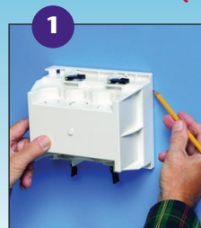
1 Using box, without trim plate as a template, mark location. Cut hole. Attach trim plate to box with supplied screws. Pull wire(s). Insert box into hole.
