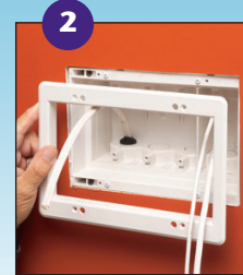
2 Attach paintable trim plate with screws provided.
