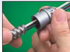
Snap onto cable and give a clockwise twist.
